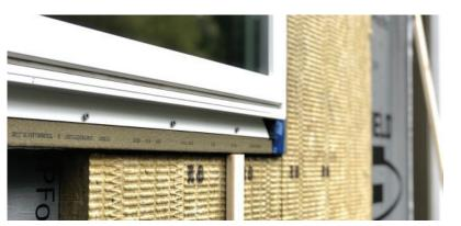
Grip-Deck® Screws attach the window flanges THROUGH the ThermalBuck™ back to the wood studs.
